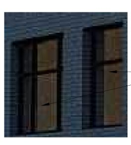
FENÊTRE HYBRIDE ALUMINIUM CHARCOAL CÔTÉ EXTÉRIEUR BLANC PVC CÔTÉ INTÉRIEUR THERMOS DOUBLE (3mm + 9mm ARGON + LOW-E + 4mm)LES FENÊTRES DOIVENT ÊTRE HOMOLOGUÉES ENERGY STAR
